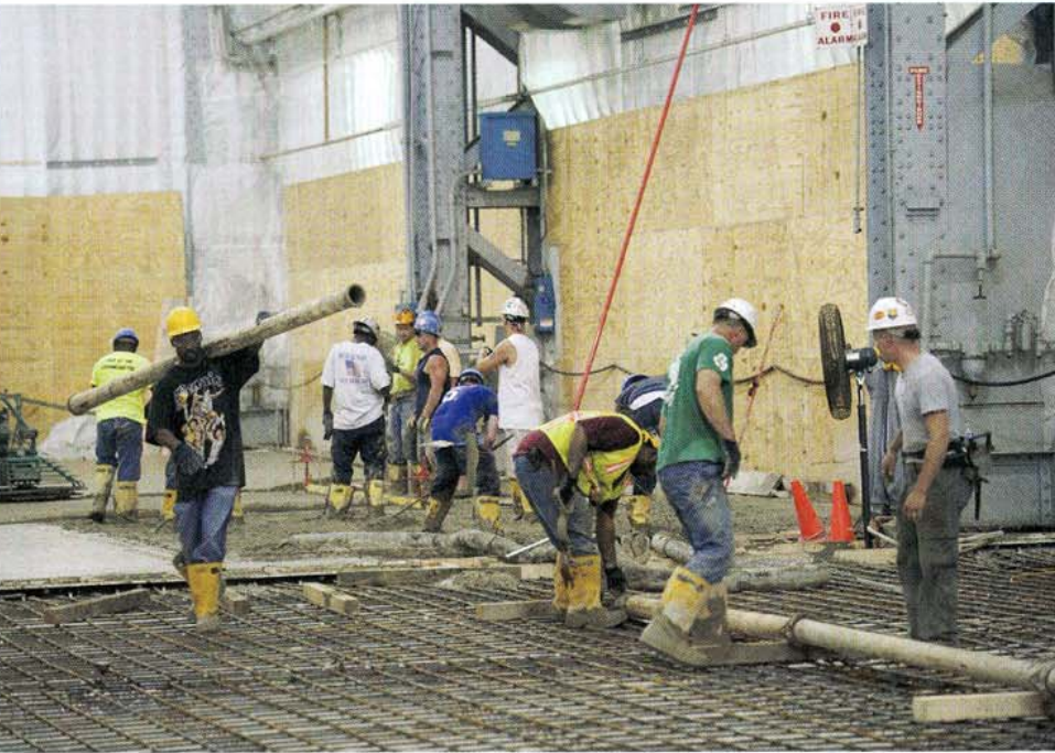
Healy, Long & Jevin crews placed superflat floors by hand using the Screed Rail from Allen Face Companies. Crews averaged FF numbers 80 percent higher than specified and FL numbers 57 percent higher than specified.
